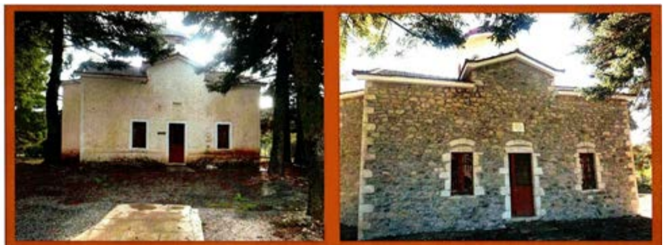
The Saint Anargyroi Chapel above, before and after the works.
